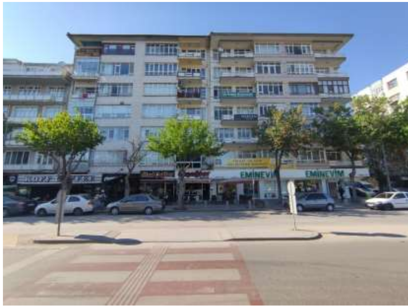
Figure 5. Güvez Apartment House Facede
