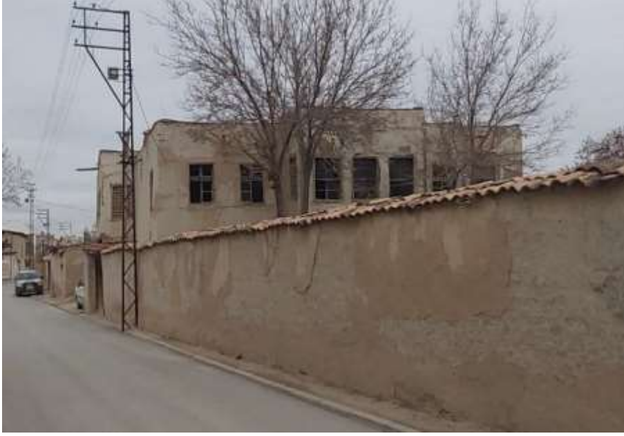
Figure 2. Nakipoğlu House Facade (Dönmez, 2021)
